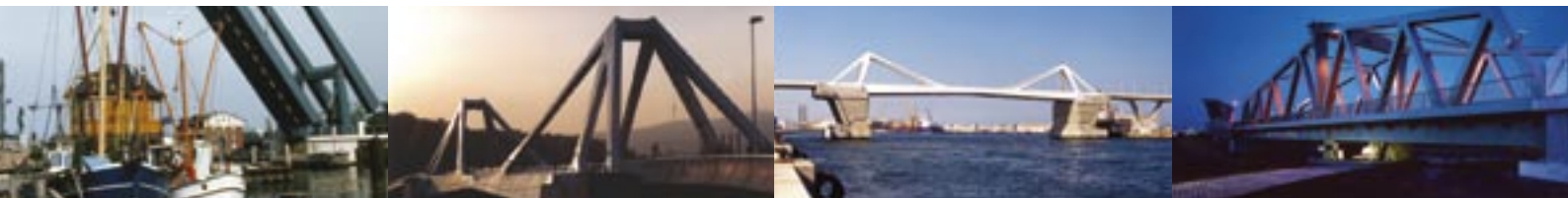
World Largest Bascule Bridge at Barcelona Harbour, Spain
